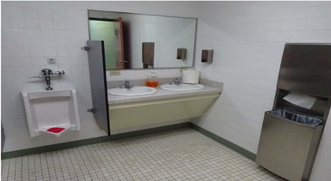
Renovation of all Men's and Women's Toilet
