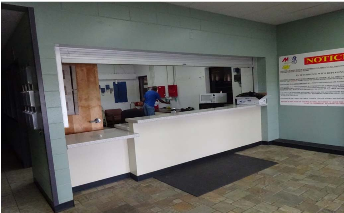
Install Solid Counter Top and Floor Tiles
