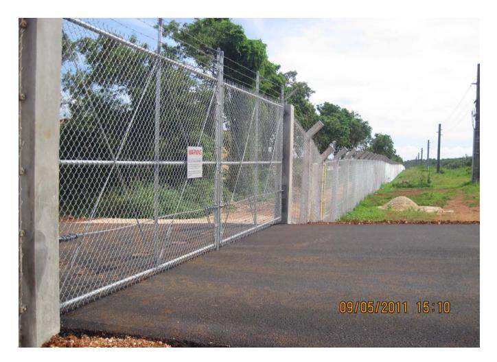
Install new ¾ inch ATFP Crash Cable 30 inches from the finish grade secured to buried 3 feet wide x 3 feet length x 4 feet deep concrete deadman anchors.
