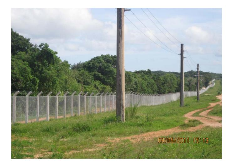
Provide and Install new additional 1500 LF of 7 feet high perimeter chain link fence. Construct 2 auxiliary vehicle access gate 24 ft in width with permanent ATFP installed equipments at locations indicated on the Plan ,new Vehicular swing gates & access gates complete with welded hinges ,can resist a max wind load of 175 mph and meets AT-FP high security requirements.
